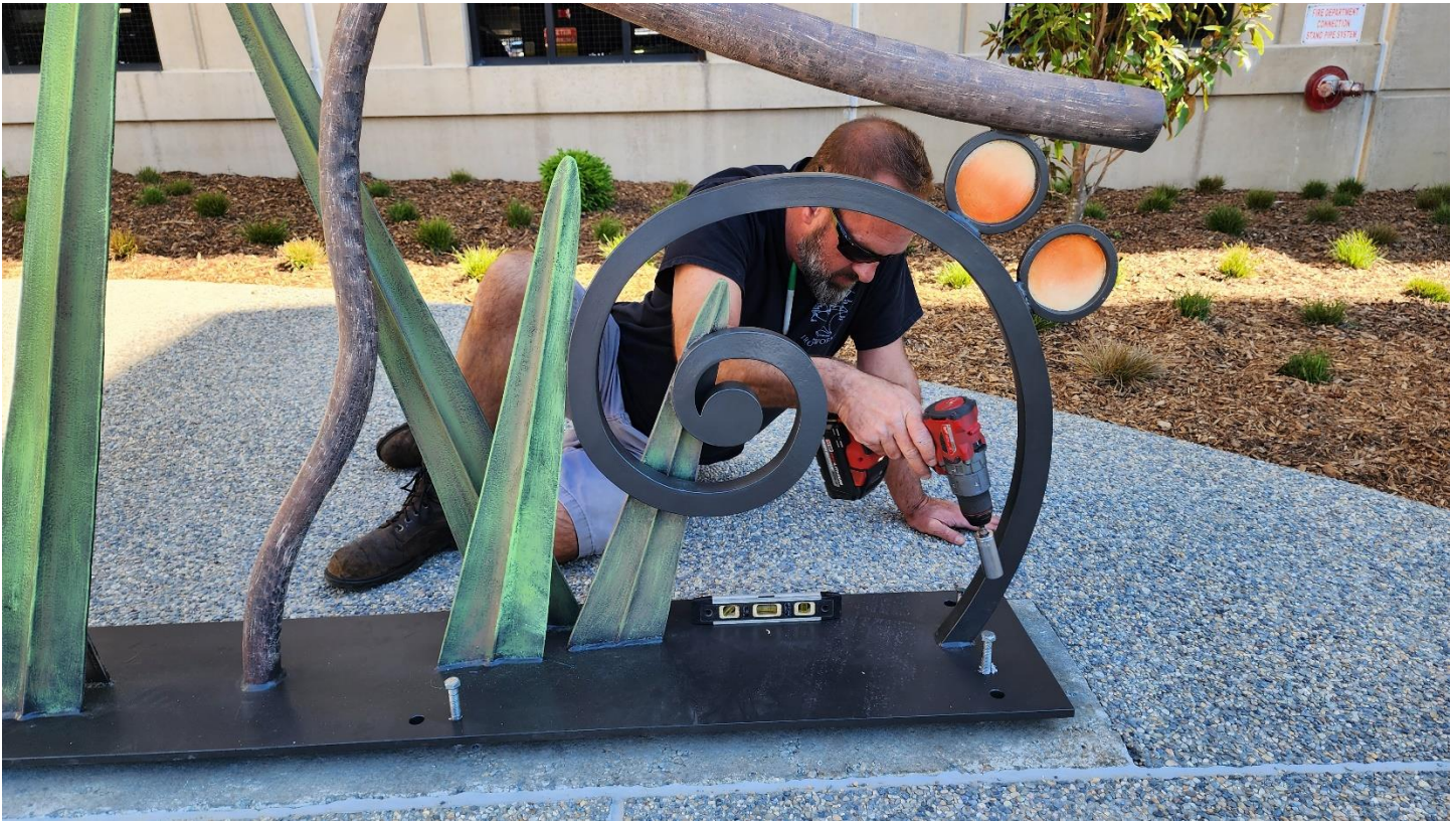
The final bolts being secured into the masonry.
